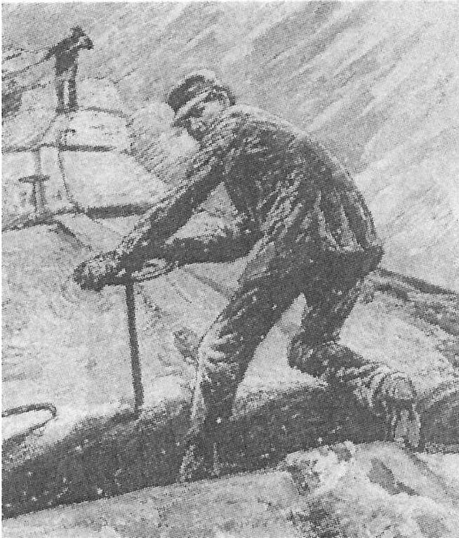
Figure 4. Trainmen manually turned a hand wheel on each car to set the brake.
